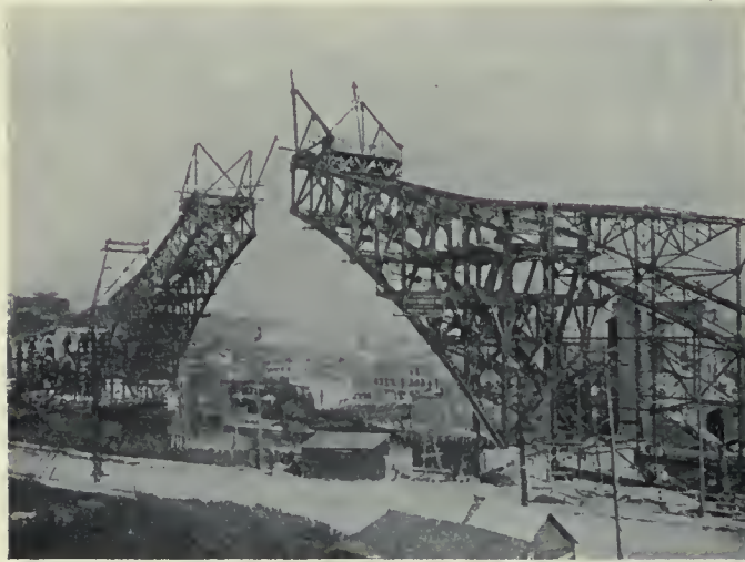
Fig. 3—Top chord Travellers lift steel from scows during erection of Cantilever.
